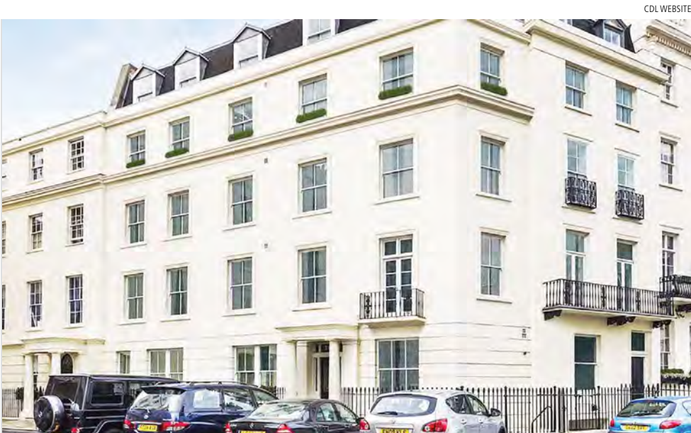
At 31 and 33 Chesham Street in Belgravia, only half of the six refurbished apartments have been sold.
