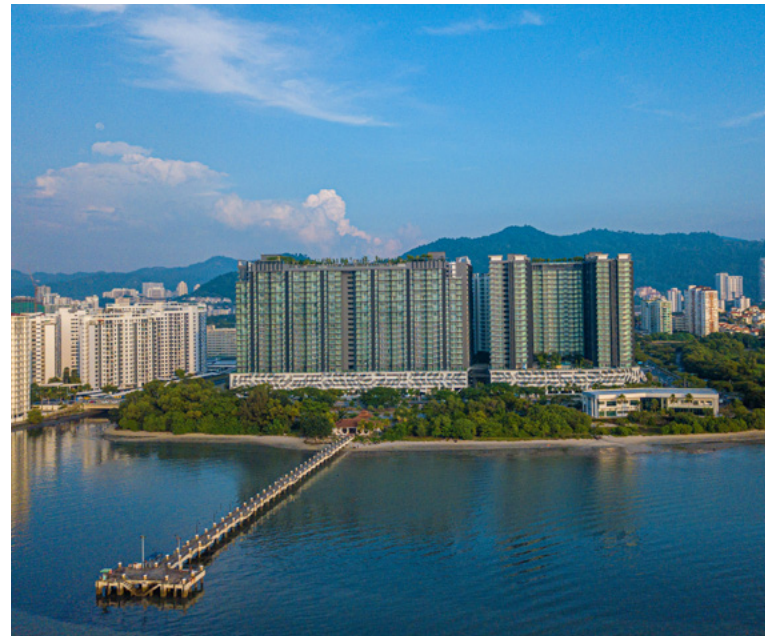
QuayWest Residence condominium in Bayan Lepas, Penang
