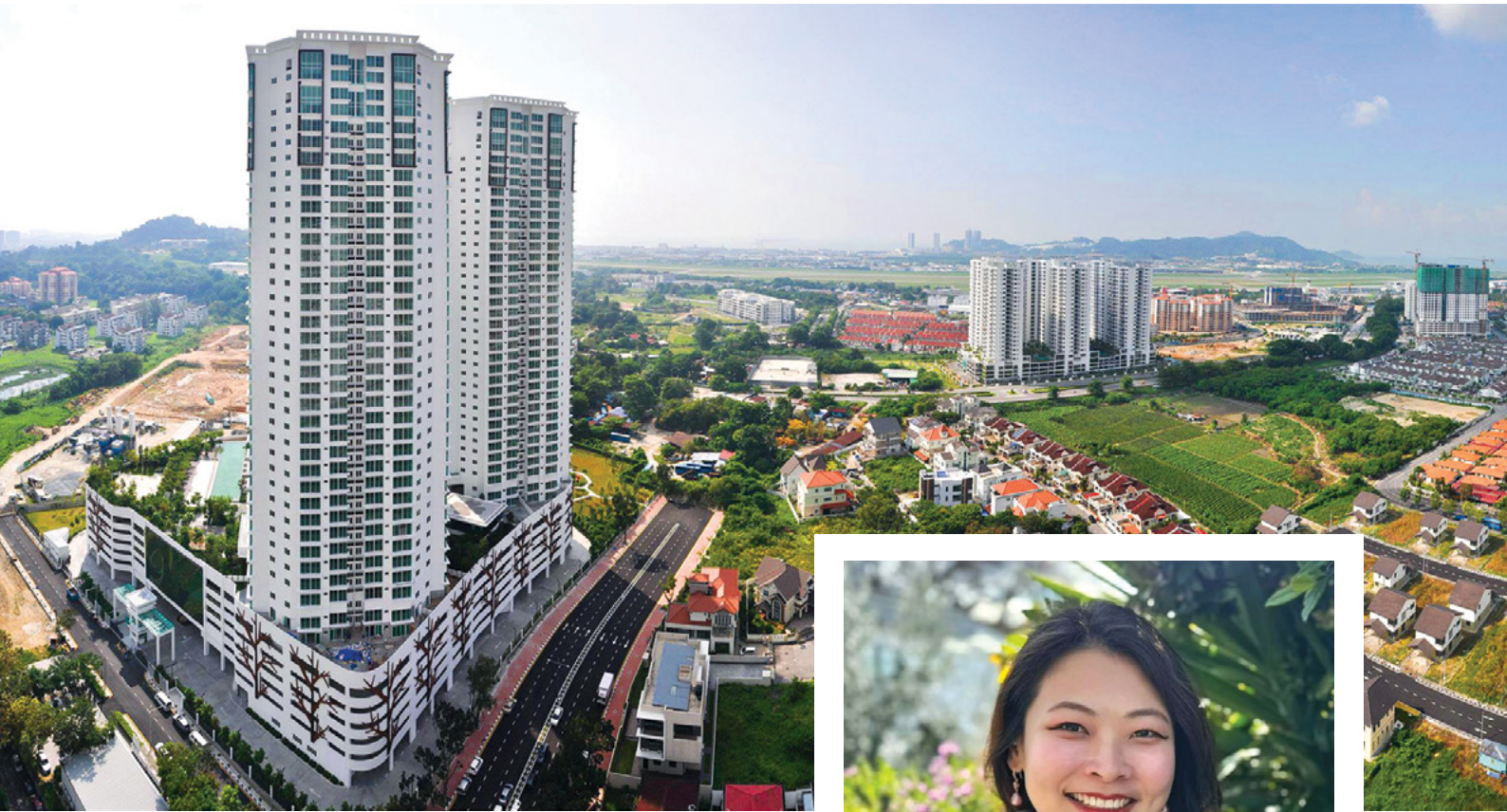
The Clovers Condominium in Sungai Ara, Penang
