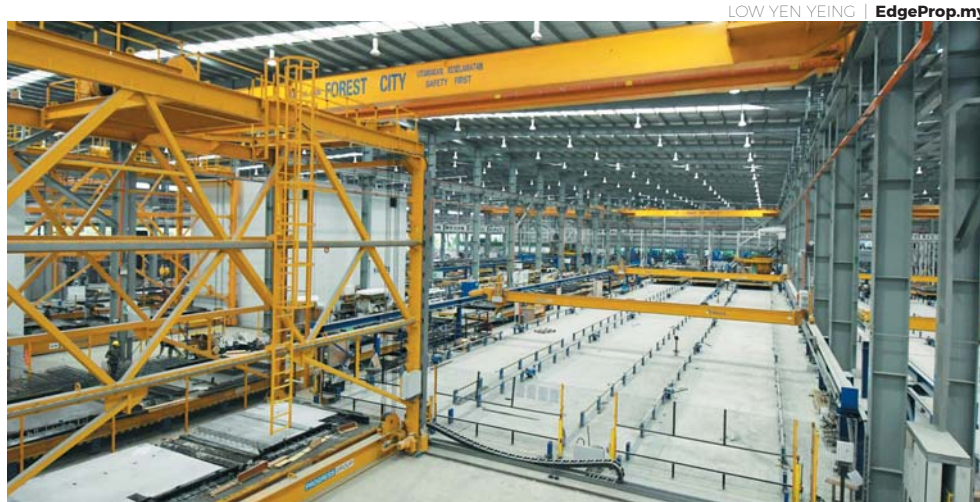
The biggest fully-automated IBS plant in Malaysia, located in Forest City in Iskandar Malaysia.
