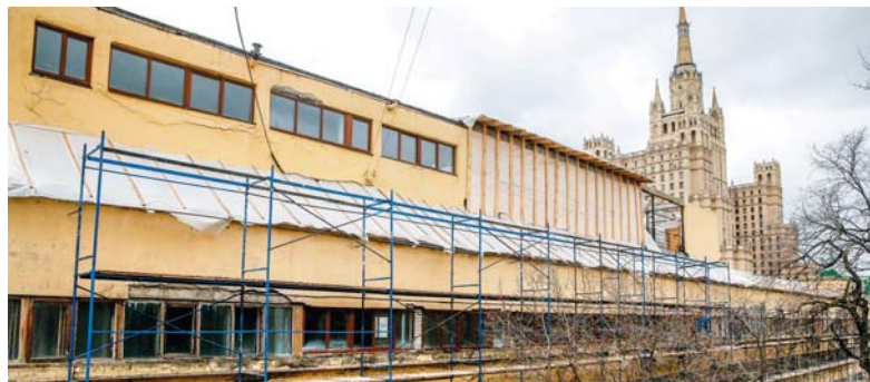
Moscow's Narkomfin apartment block is finally being restored to its original pioneering state in the middle of the Russian capital.
