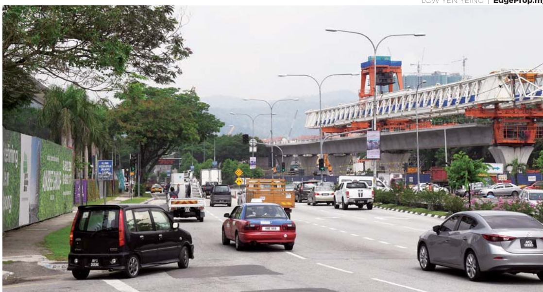
One of the MRT stations that is coming up in the area, across the road from the upcoming Unio Residence, KL North.
