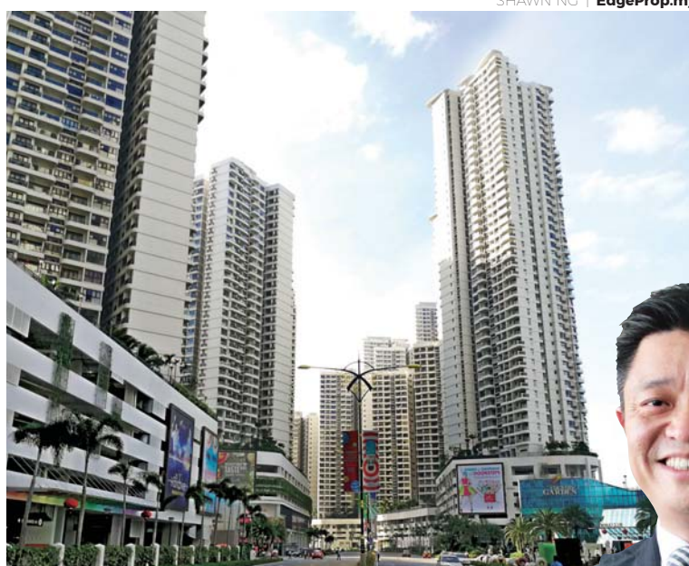
Country Garden Danga Bay is Country Garden Malaysia's first development in Malaysia.
