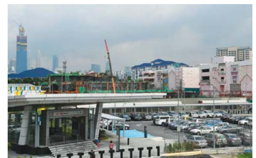
The renovation works of AEON Maluri will be completed end-2019.
