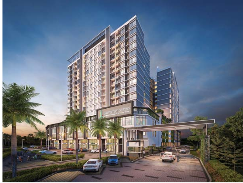
Amverton Greens comprises 280 units with built-ups ranging from 953 sq ft to 1,528 sq ft.
