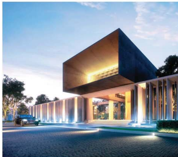
The modern clubhouse at Grandezza.
