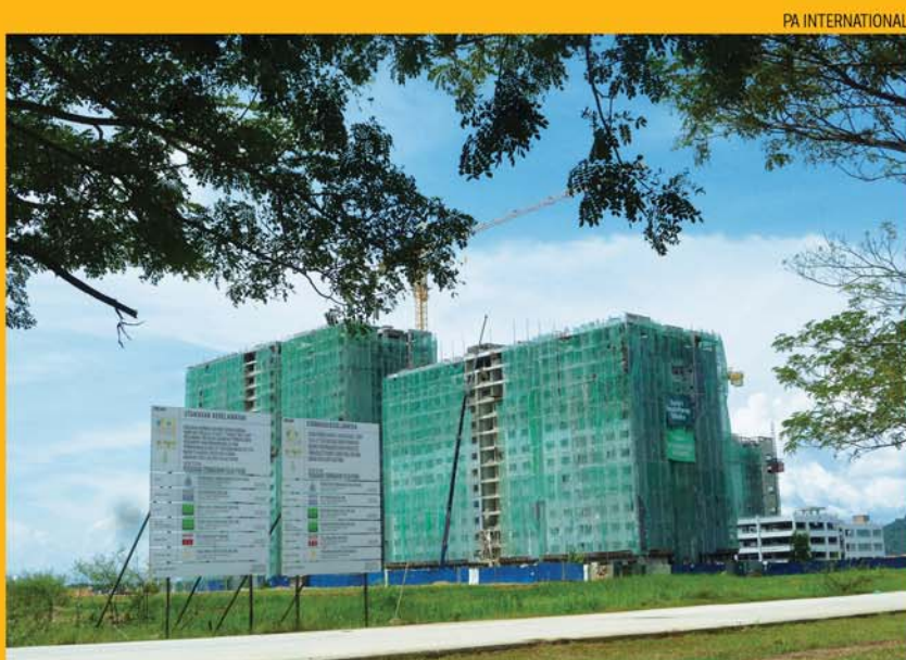
Bandar Cassia's Suria 1 affordable homes are nearing completion.
