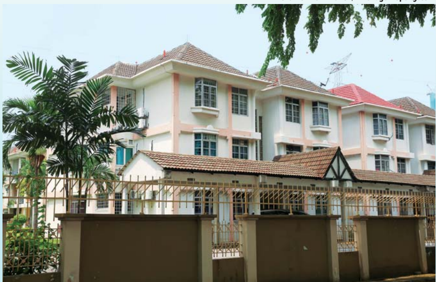
Taman Maluri is one of the oldest housing areas in Cheras KL
