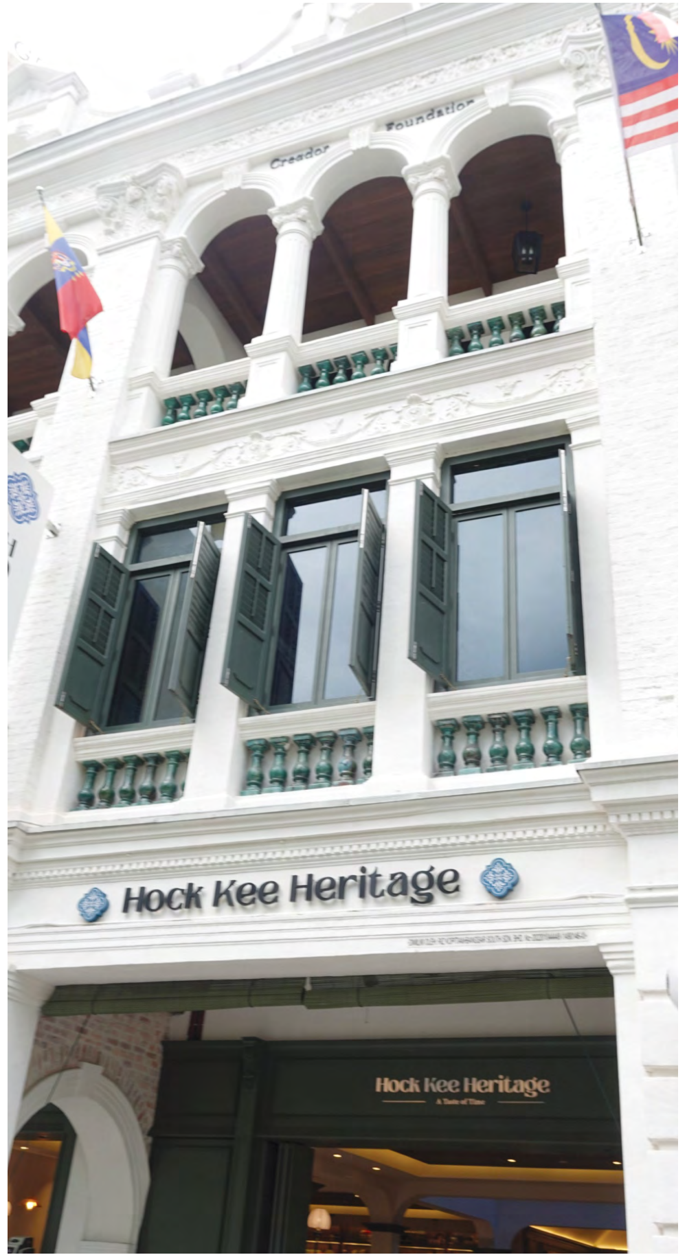
Hock Kee Heritage cafe operating within a restored shophouse in Medan Pasar, reflecting the adaptive reuse of KL’s historic commercial buildings
