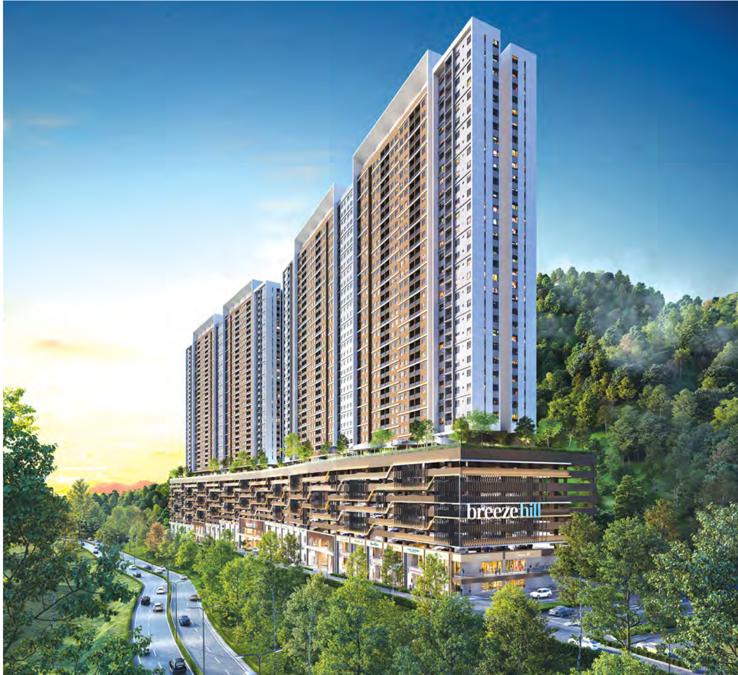
Sited in Gohtong Jaya, Breeze Hill is a defining address within Tropicana WindCity, a 596-acre master-planned township — the first of its kind in Genting Highlands.
